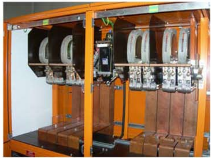
Mechanically Latched Bar Mounted 4000A Contactor
